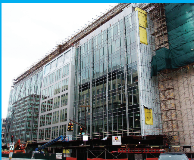
Koch Institute construction progress as of September 2009.
