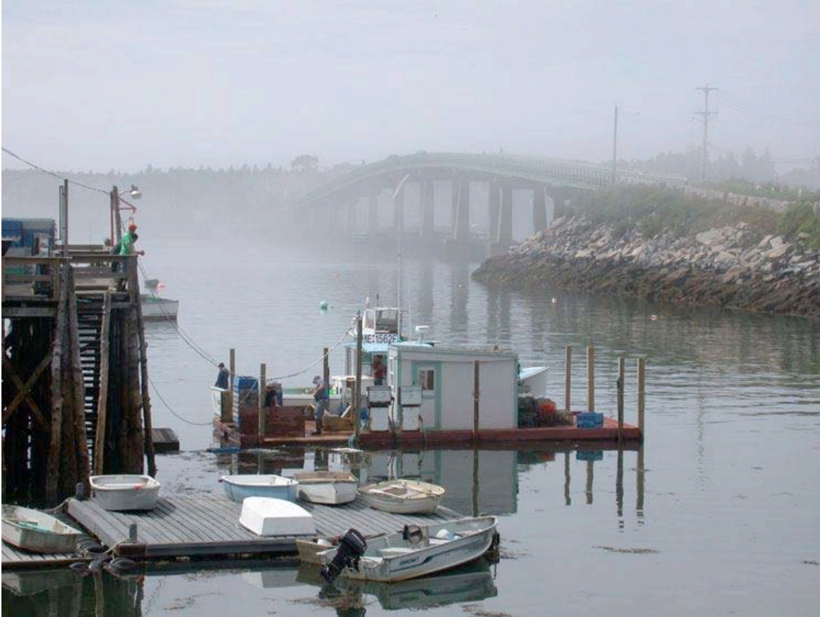
Beals Island Bridge
