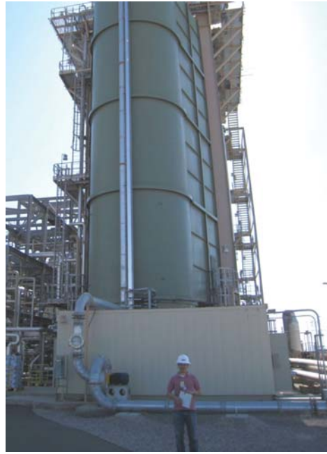
APS Red Hawk Power Plant Field Test
