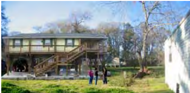
The site with the future LiftHouse
