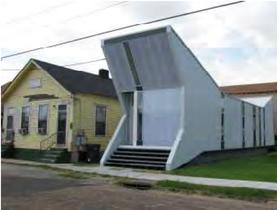
Alligator House by buildingstudio
