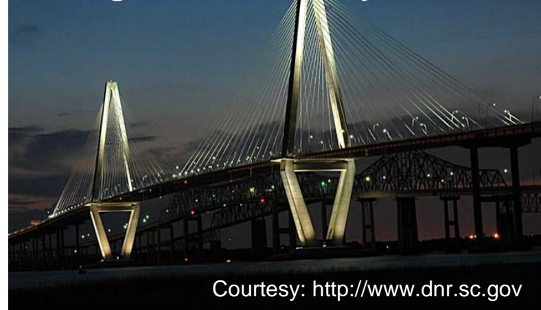
SCDOT: Bridge on Cooper River Design-Build Delivery Method
