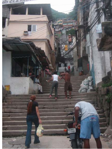
Figure 9. The main “street” in Santa Marta is a set of stairs which narrows from the base, shown here. The lowest steps on the hill are concrete. The sand bags on the right are being used to make steps farther up the hill.
