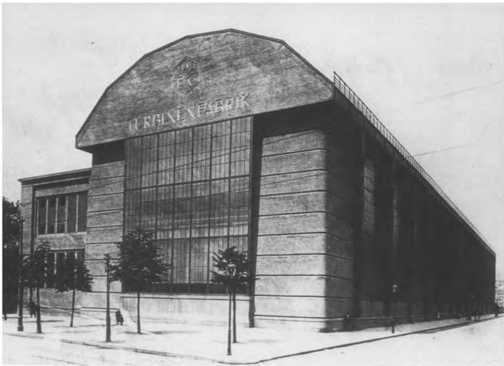
11. Behrens, AEG Turbine Factory, Berlin, 1909, view of two principal façades
