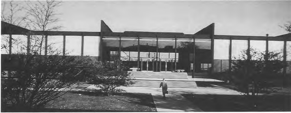
37. Mies, Crown Hall, Illinois Institute of Technology, Chicago, 1956
