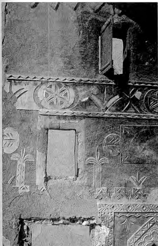
FIGURE 5. Unaizeh, Saudi Arabia. Indigenous mud brick building. (Photo by author.)
