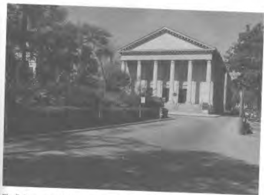
Fig. 7. Savannah, Chippewa Square in Brown Ward, 1733. First Baptist Church (Elias Carter, ca. 1833).
