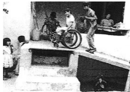
This ramp in a Mexican village clinic was built in a very limited space. The board over the steps lifts out of the way, so that people can use the steps when the ramp is not needed.
