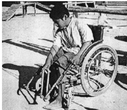
To move from wheelchair to walker, Carlos first lifts aside the footrest. (A single footrest for both feet, hinged on one side, makes this easier for him.)
