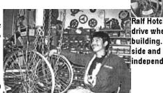
Ralf Hotchkiss examines the one arm drive wheelchair which Martin is building. The 2 hand-rims are on one side and can be powered together or independently with one hand.
