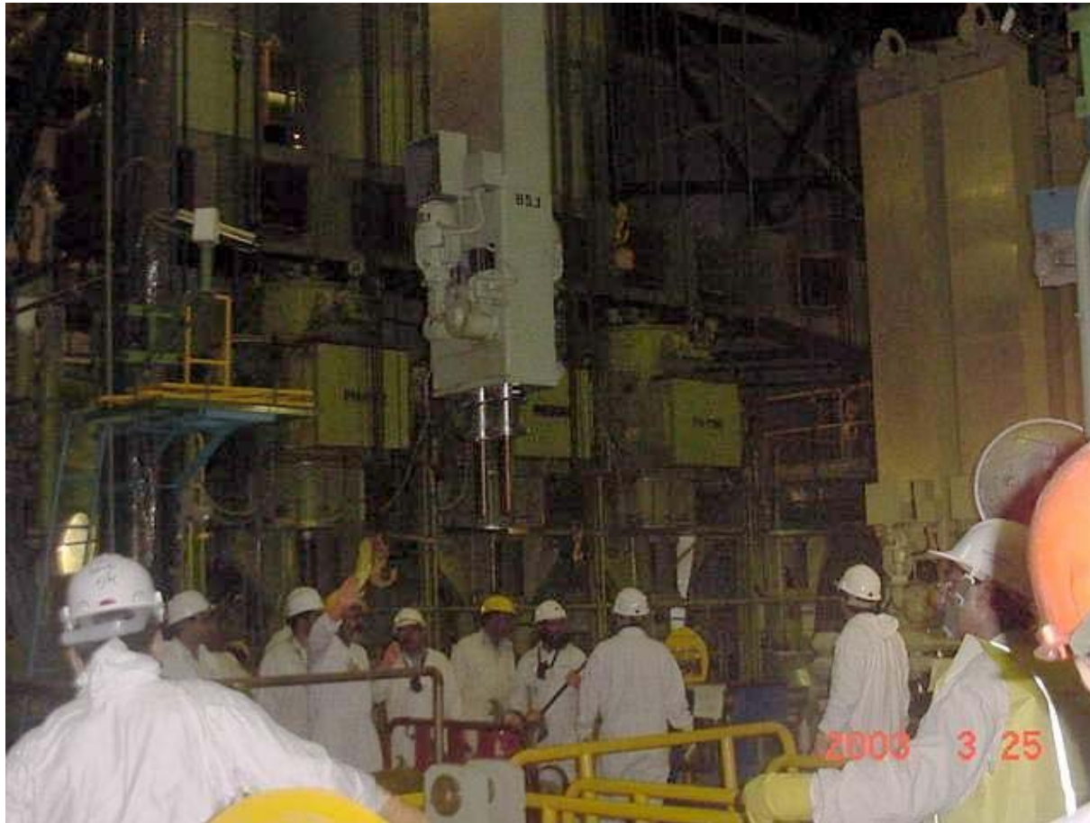
Reactivity Drive Mechanism is being transferred to its parking position
