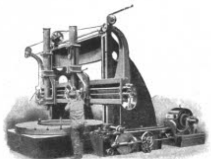
14-INCH BORING AND TURNING MILL, ELECTRIC DRIVE.
