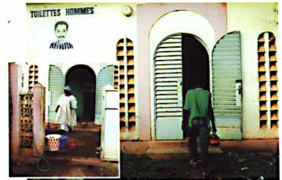
Water kiosk and toilet facilities in a neighborhood market
