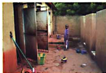
SEMA SANIYA public toilets are used 200 times every day of the workweek
