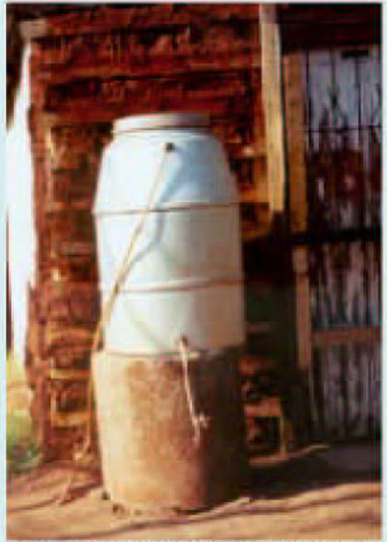
A semi-pressure system with a ground tank.
