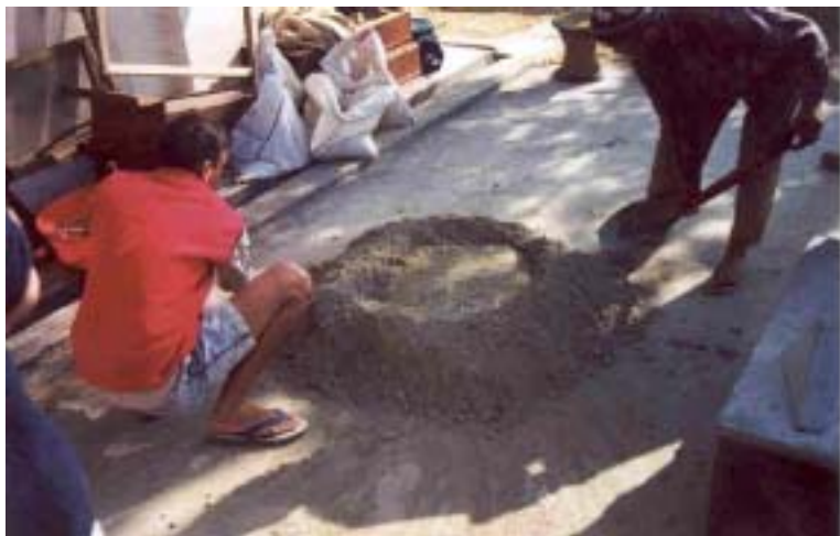
Figure 50 - Concrete Mixing II
