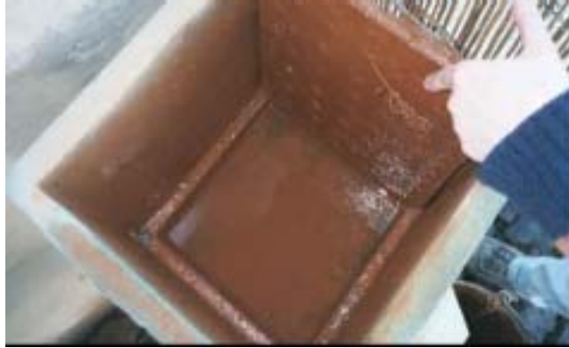
Figure 31 - Iron Rust Deposit on Top of the Fine Sand Layer
