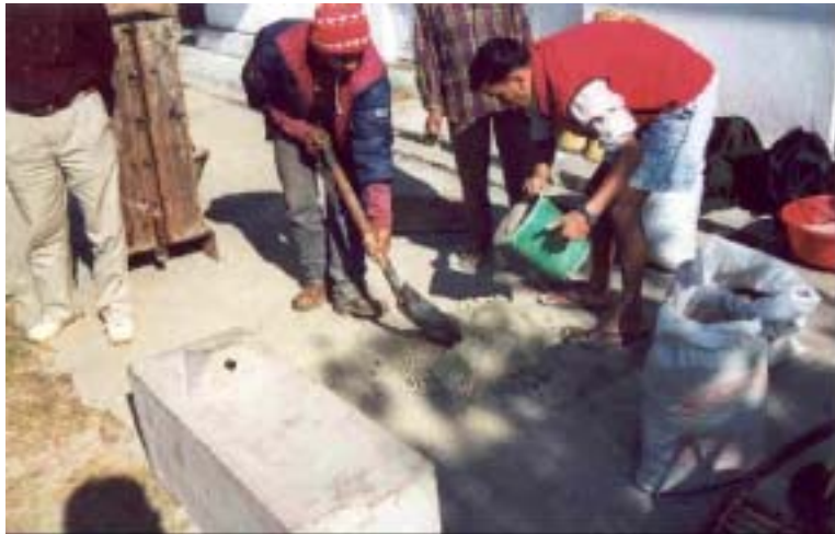
Figure 49 - Concrete Mixing I
