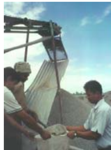
Figure 12 - Filling up Bags of Crushed Sand
