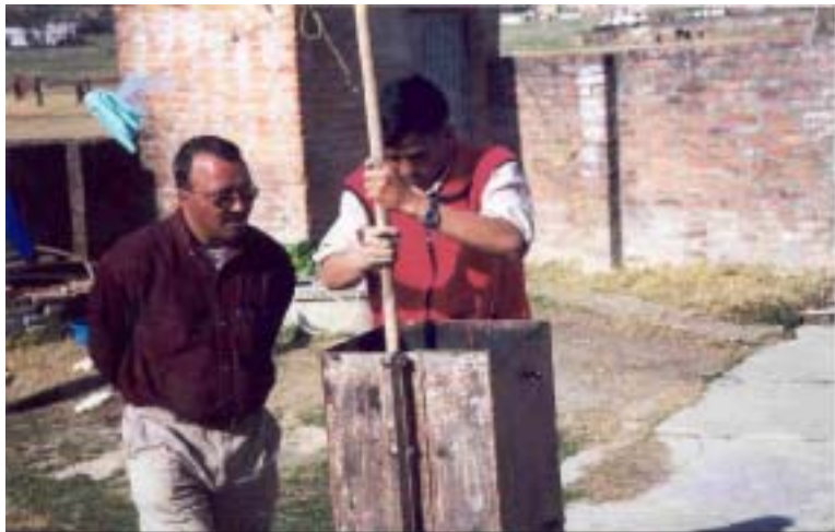
Figure 51 - Tamping the Concrete Mixture with a Wooden Rod
