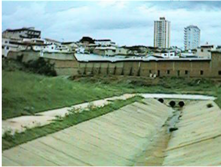
Figure B-2: Storm water channel, image taken at the source of the Jardim de Boa Esperança stream
