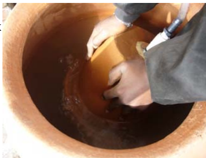
Figure 6-7 Leak Testing Completed KWK
