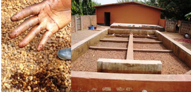
Figure 14 Mafi Kumase HRF: dirty gravel media (left) and view of HRF from the inlet (right)
