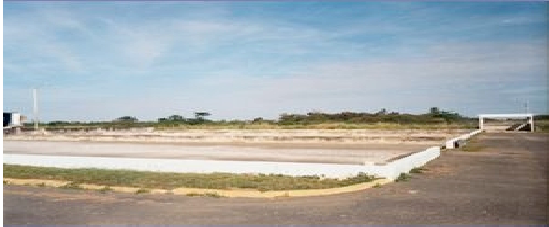
FIGURE 22-SAND DRYING BEDS IN VEGA BAJA PLANT
