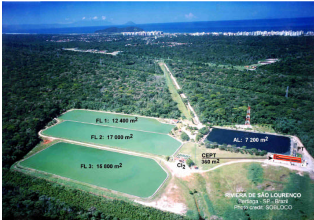
Figure 1-5: CEPT treatment implemented at Riviera de São Lourenço (Source: Sobloco Construction Company, http://www.sobloco.com.br )
