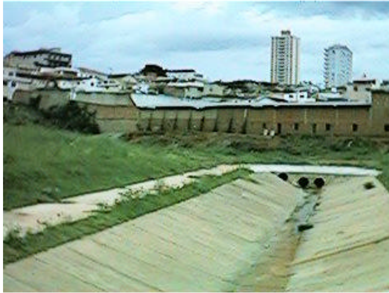
Figure 3-2: Storm water channel, image taken at the source of the Jardim de Boa Esperança stream
