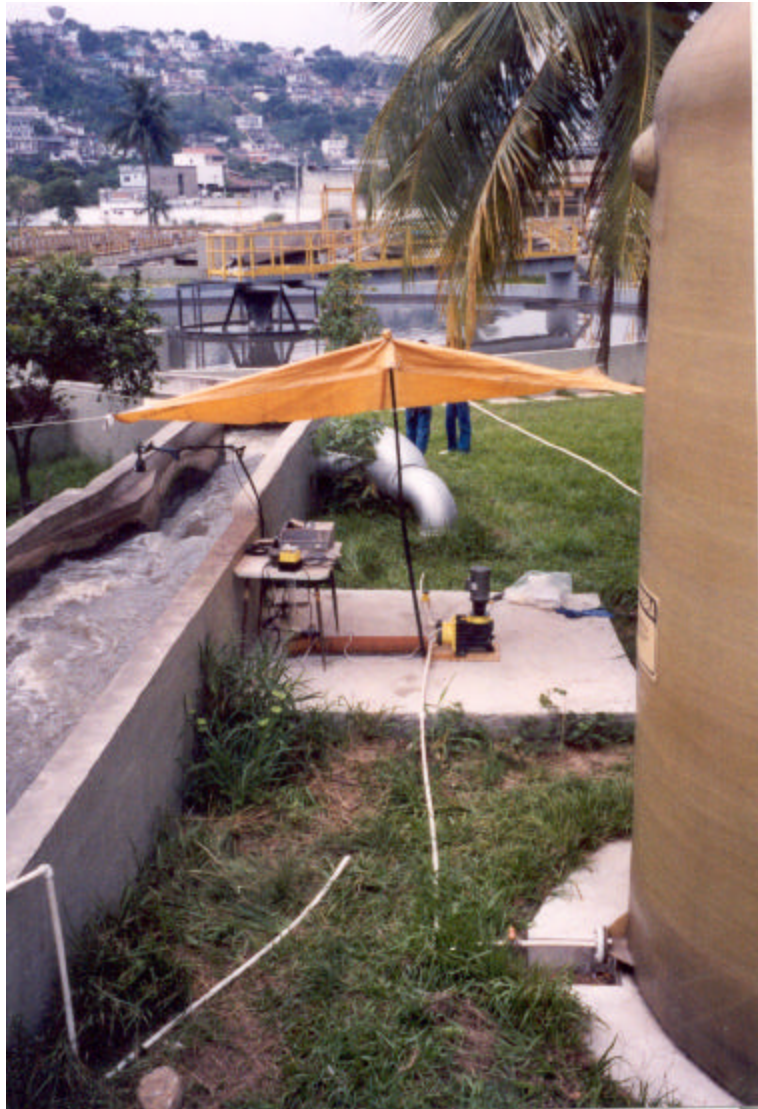
Figure 1-8: Detail of the pilot-plant chemical dosing system at Ipiranga (Source: Susan Murcott)
