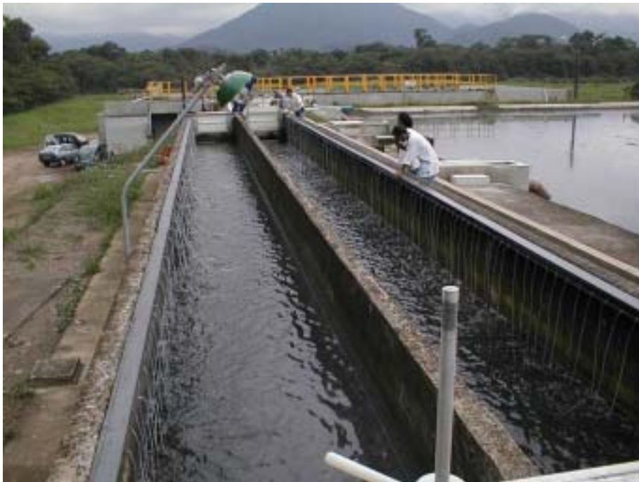
Figure 8-4 Flocculation and CEPT Tanks and Lagoon at Riviera
