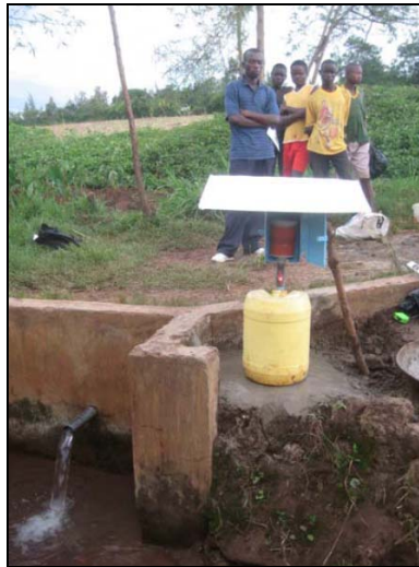
Figure 7: The RWP Installed Chlorine Dispenser in Kenya (Berens and Van Dusen 2007)
