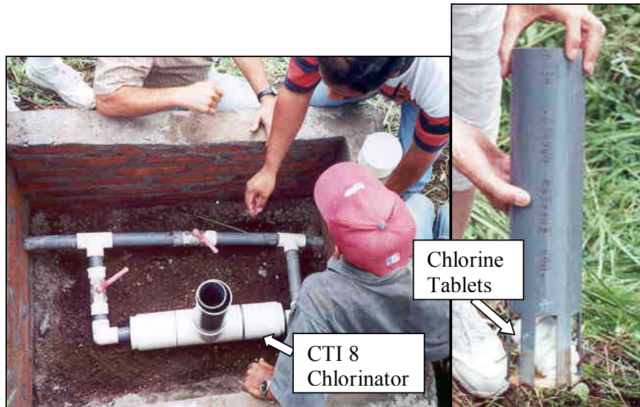
Figure 10: CTI-8 Chlorinator Installed in Nicaragua (Yamana and Nepf 2003)
