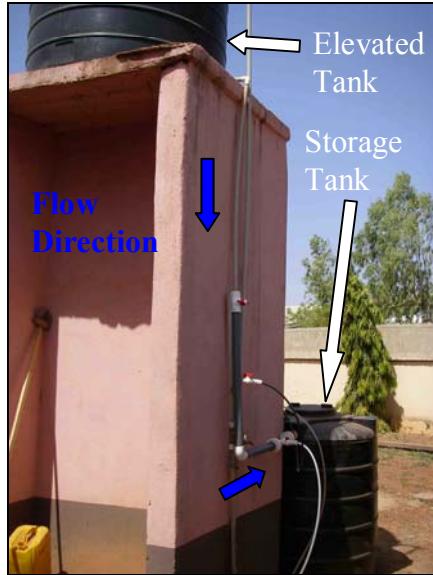
Figure 35: Configuration and Flow Direction of System
