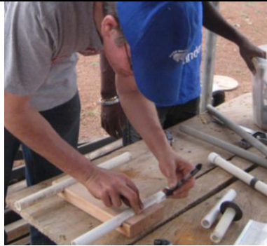
Marking where the wood hits the PVC pipe to indicate where to add friction tape
