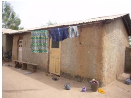
One Compound Structure
