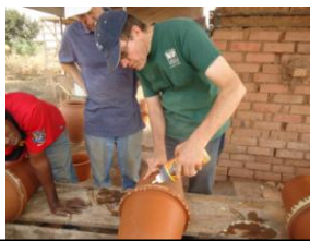
Re-applying glue to leaking spots
