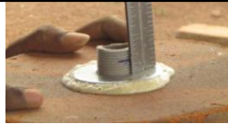
Measuring out exact height for PVC riser pipe
