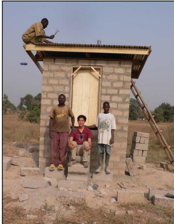
Figure 7-2 The finished structure with the construction team
