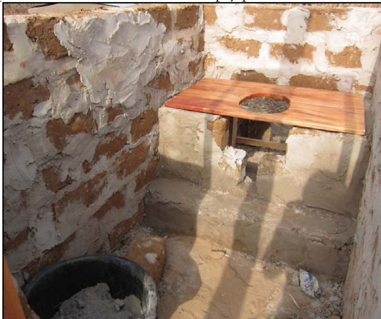
Figure 7-4 Interior of latrine structure in mid-construction (Photo credit: Mette Andersen)
