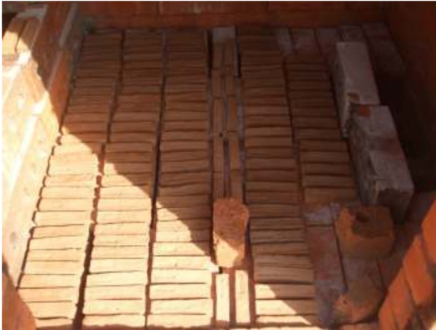
Figure 4-7: Loading of Clay Beams
