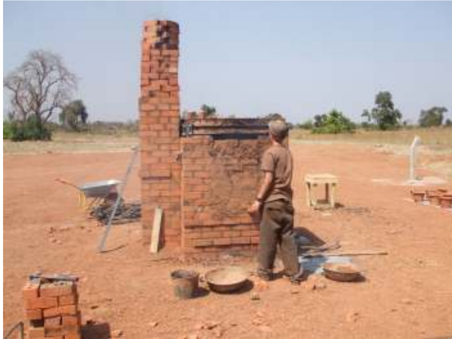
Figure 4-5: Downdraft Mani Kiln, Showing Mortar-Sealed Door (Photo Credit: Leah Nation, 2010)
