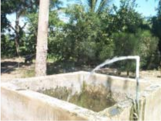
Figure 7 Examples of a free flowing captage (Dumay 5) and a fauceted captage (Bas Limbe 2).
