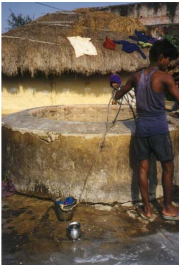
Figure 2-10: Typical Hand Dug Well
