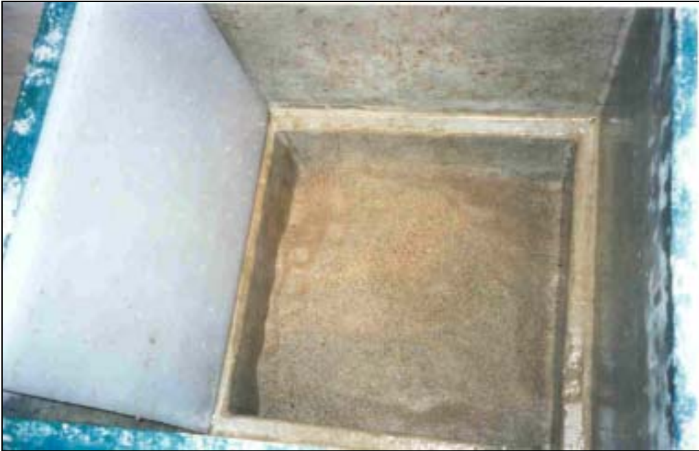
Figure 36: Water level at rest below top layer of fine sand.
