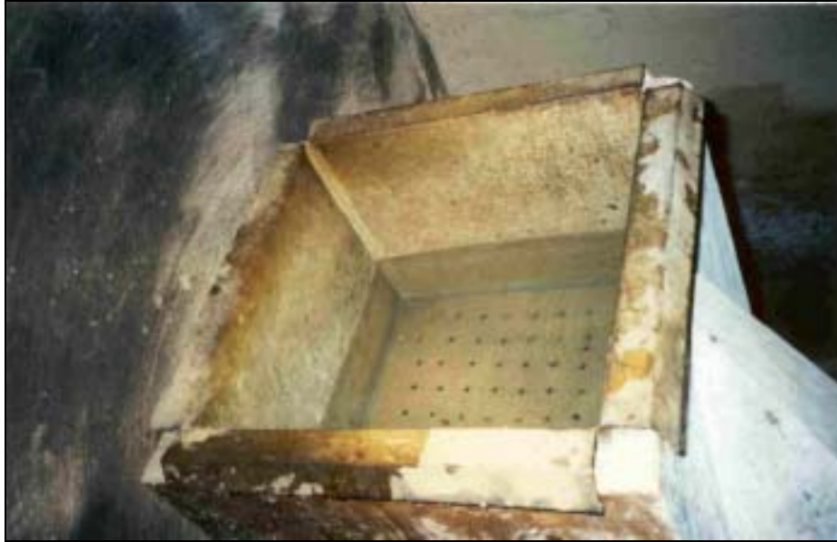
Figure 19: A metal pot used as a diffuser basin in a round BSF
