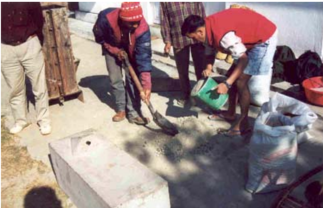
Figure 12: Concrete Mixing I
