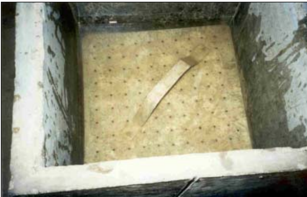
Figure 15: A typical metal diffuser plate with handle in Nepal
