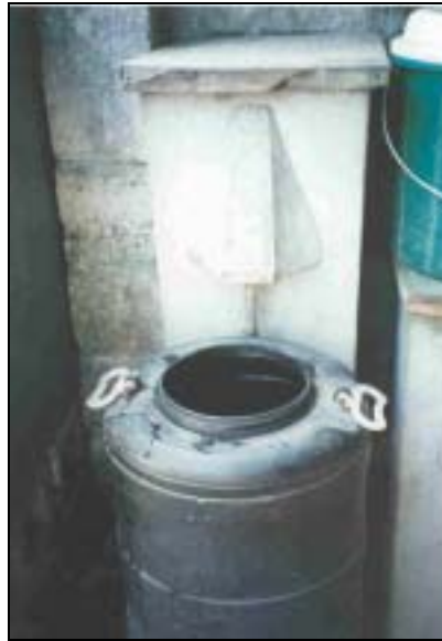
Figure 33: Spout is not plugged, allowing continuous flow.
