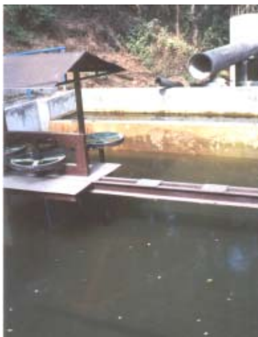
FIGURE 3-4: OFFLINE FLOCCULATION TANKS AT BALAJU.
