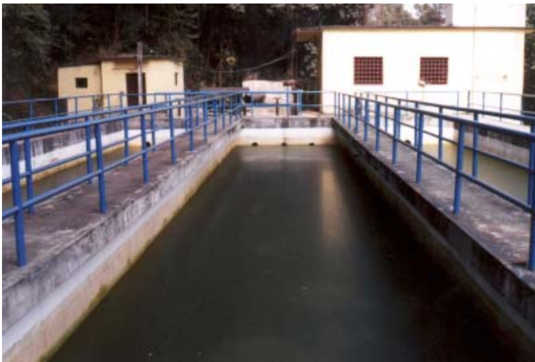
FIGURE 3-5: OFFLINE SEDIMENTATION BASINS AT BALAJU.
