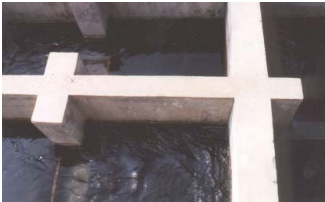
FIGURE 3-2: CLOSEUP OF WALLS IN FLOCCULATION BASIN AT MAHANKAL.
