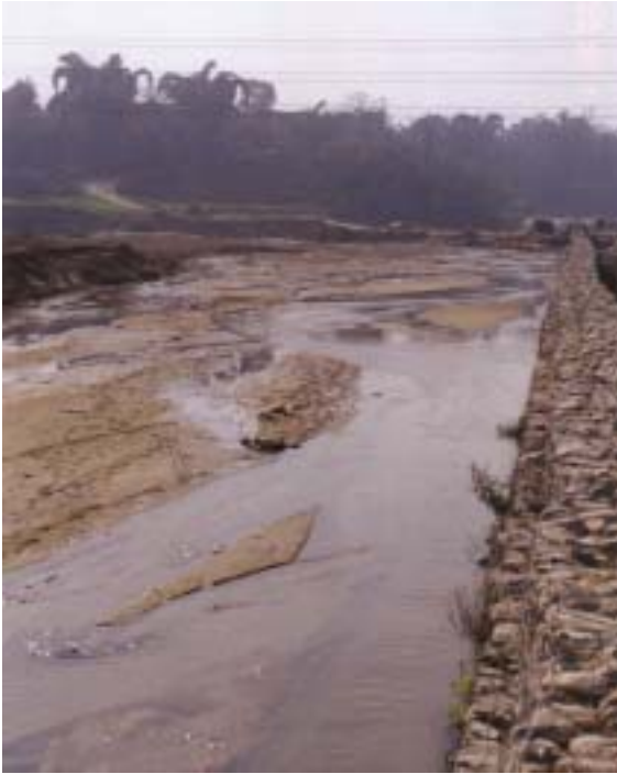
Figure 22: Picture of gabion blocks
