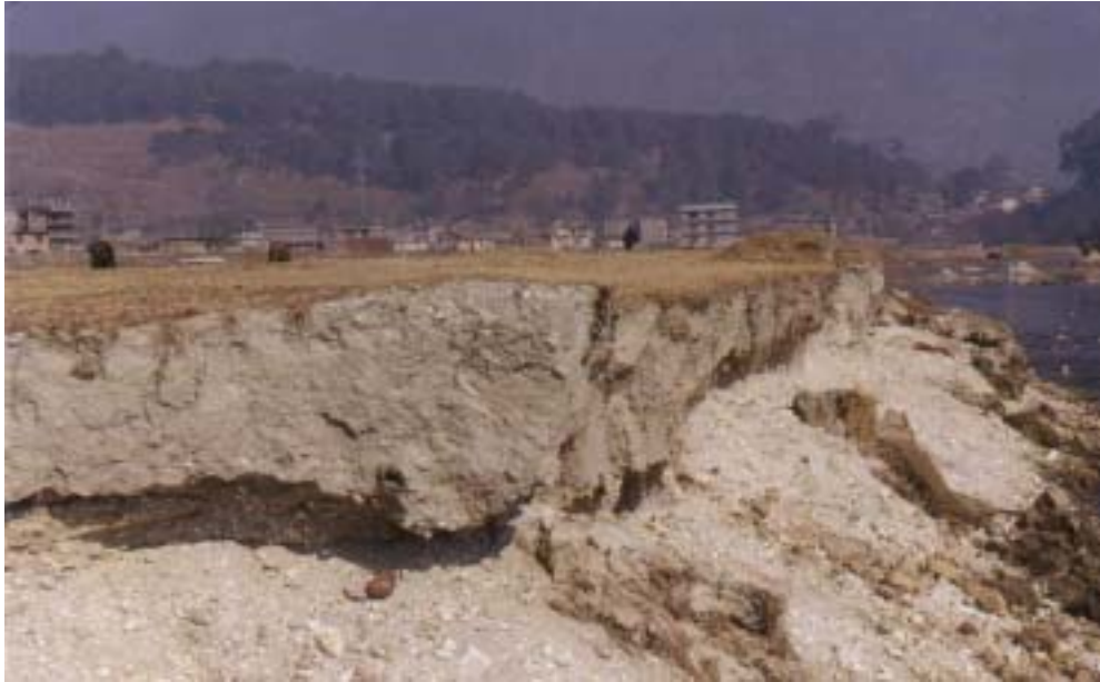
Figure 20: Picture of river bank erosion near Gokarna
