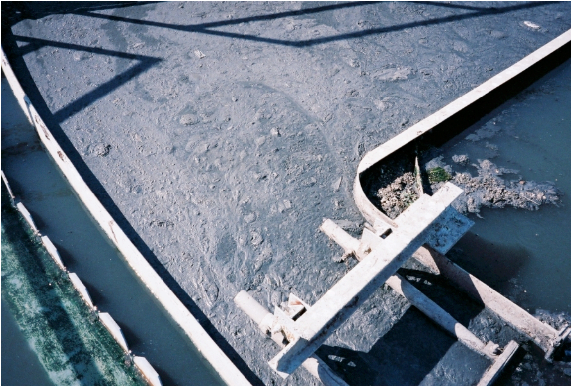
Figure 6: Floating sludge at Vega Baja
