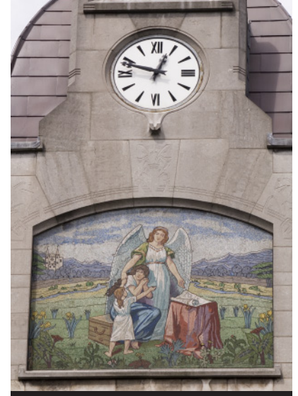
The tiled façade of the Greenpeace Building (opposite)
