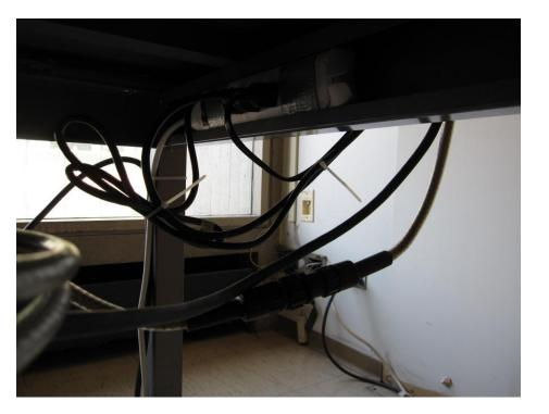
Finding 2 44506: ES-1 Extension cords were not used properly (e.g., daisy chained, used in place of permanent wiring). (Electrical Safety)
