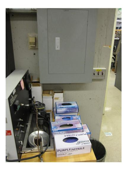
Finding 3 44507: ES-4: Access to an electrical panel was obstructed. (Electrical Safety)
