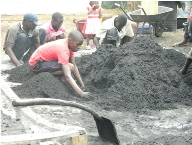
12. To ensure binder gets well absorbed they further mix with hands
