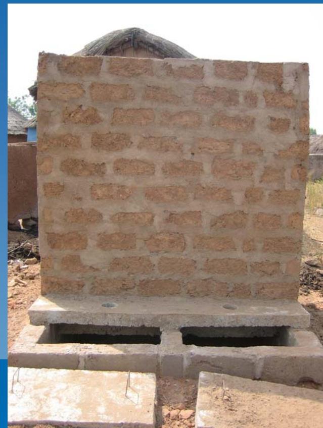
Latrine in the process of being built
