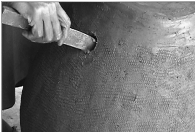
Figure 7-3: Tap opening widened using a kitchen knife.
