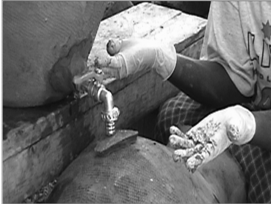
Figure 10-7: Tap attachment. Tap is fixed in place using nill on inside and outside of vessel.
