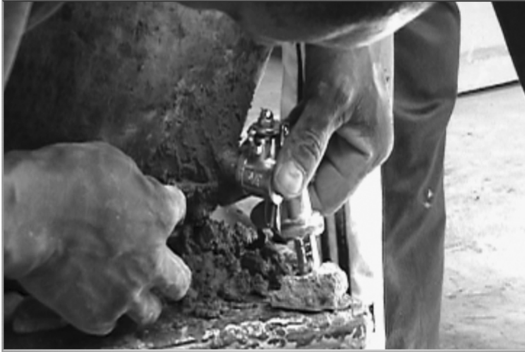
Figure 10-11: Tap attachment. Stabilization tap using cement.
