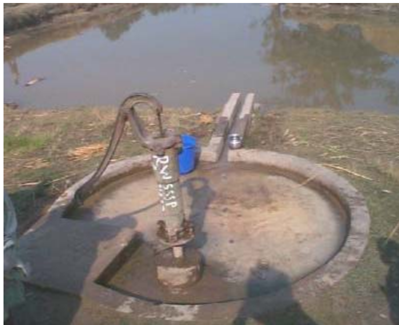
Figure 2 A Typical Suction Tubewell
