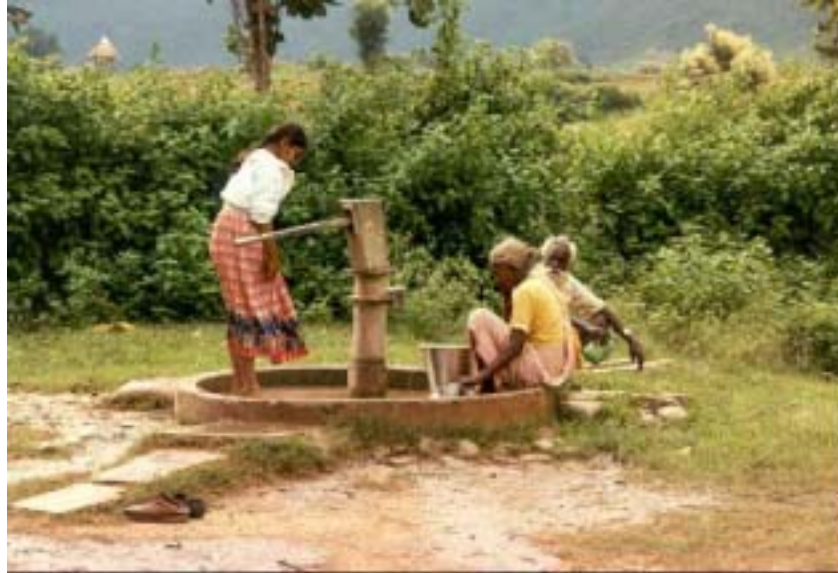
Figure 1 A Typical Lift Tubewell
