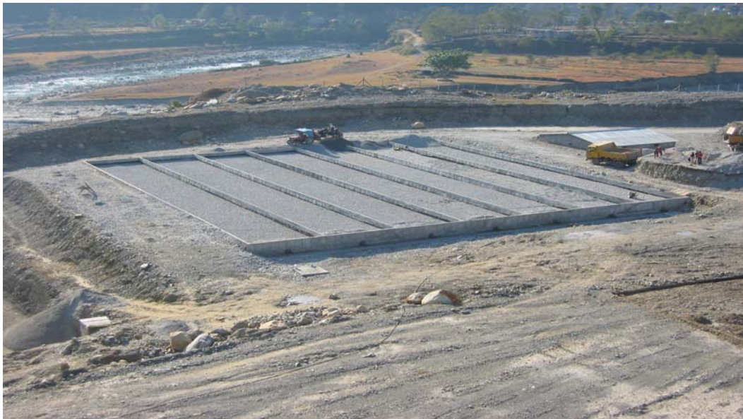
Figure 5.16: Sand Drying Bed
