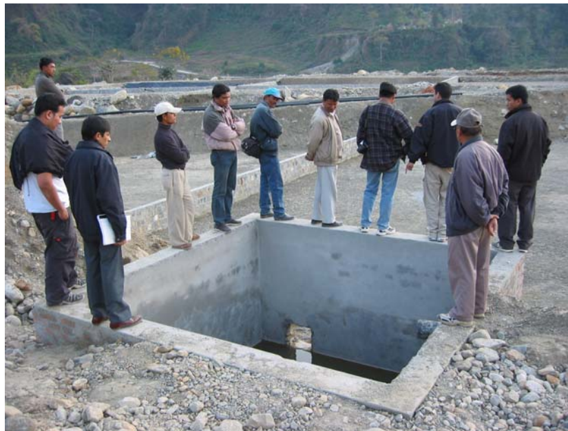
Figure 5.18: Intermittent Feeding Tank for Horizontal Bed.
