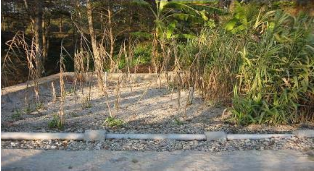
Figure 5.8: Horizontal Flow Bed at SKM Hospital
