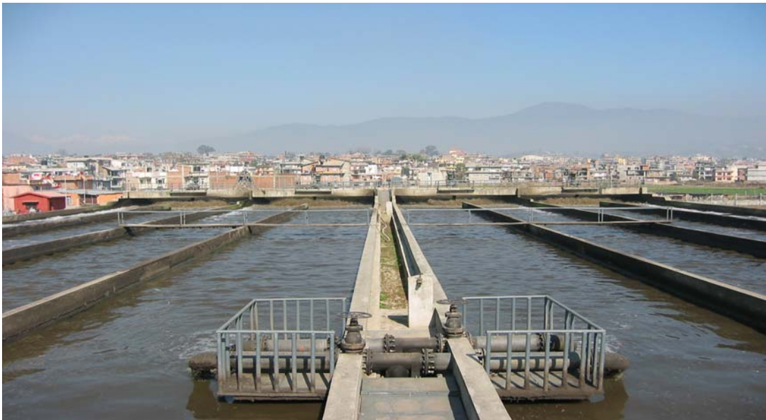
Figure 2.3: Guheshwori Wastewater Treatment Plant.
