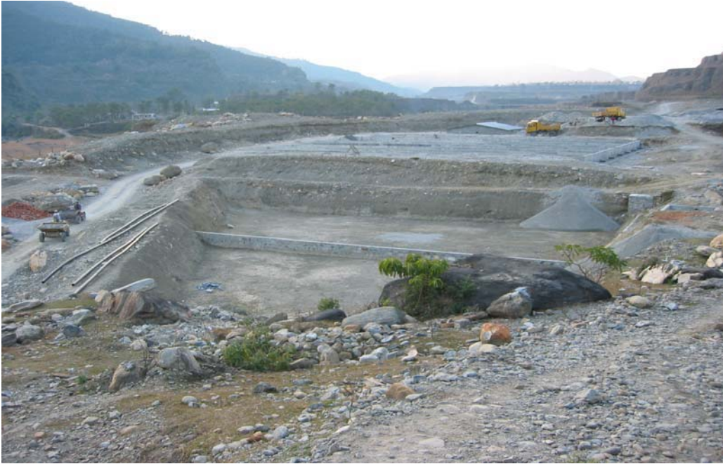
Figure 5.19: Horizontal Flow Bed
