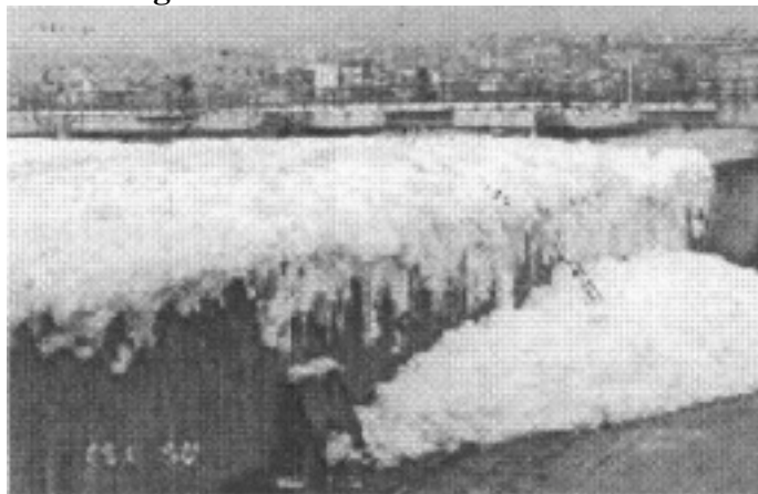
Figure 3.1: Foaming in the oxidation ditches at Guheshwori WWTP 11
