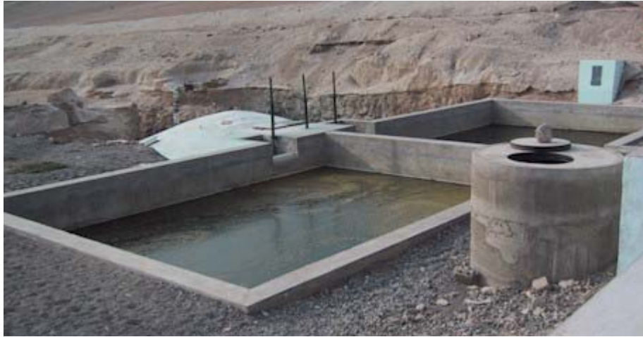
Figure 6.14: Fine Sand Bed (Covered with Water)
