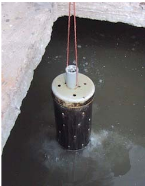
Figure 6.4: CBV Treatment Plant – Chlorine Diffuser in Last Tank
