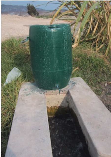
Figure 6.7: Barrel Containing Aluminum Sulfate Solution
