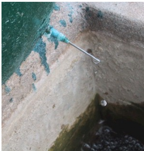
Figure 6.8: Adding Alum Drop by Drop to Influent Water
