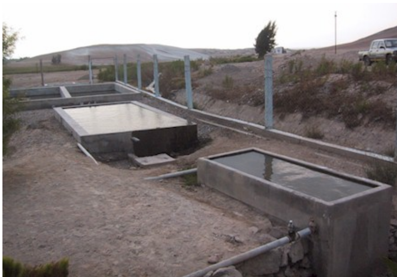
Figure 6.6: El Triunfo Pre-Treatment Tanks
