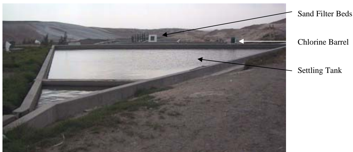
Figure 6.10: Coagulation & Settling Tanks in the Foreground and the Pre-Chlorination Tank & Sand Filtration Beds in the Background
