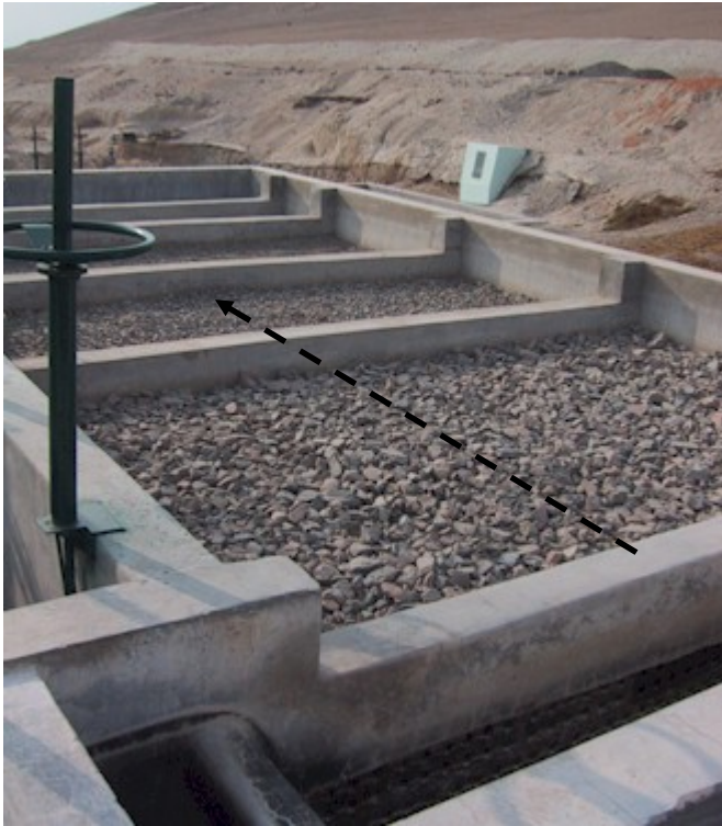
Figure 6.12: Gravel Beds (Dashed Line Indicates Direction of Water Flow)
