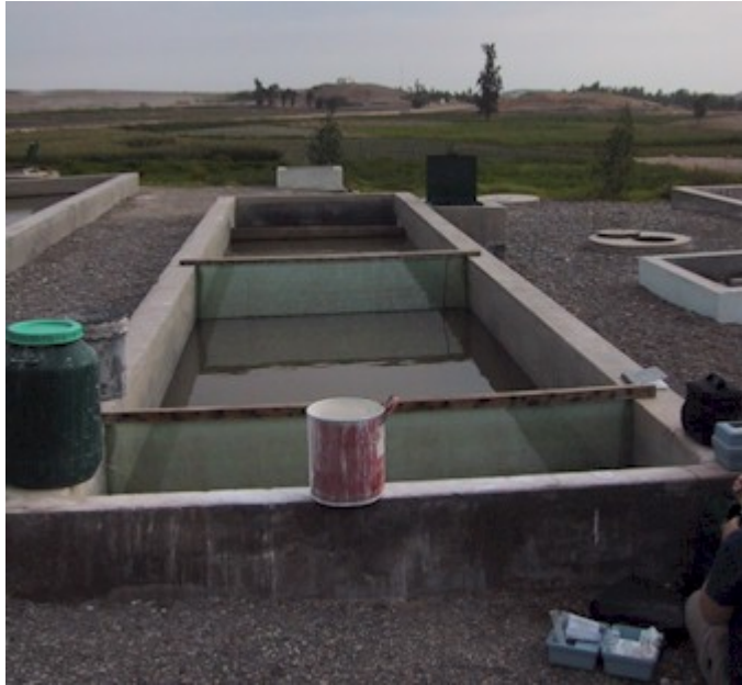
Figure 6.11: Pre-Chlorination Tank with Chlorine Barrel (Left Foreground)
