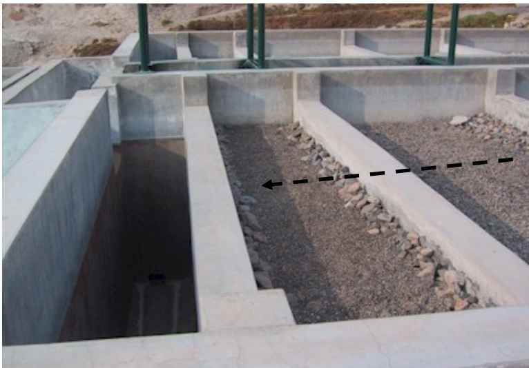
Figure 6.13: Fine Gravel & Coarse Sand Beds
