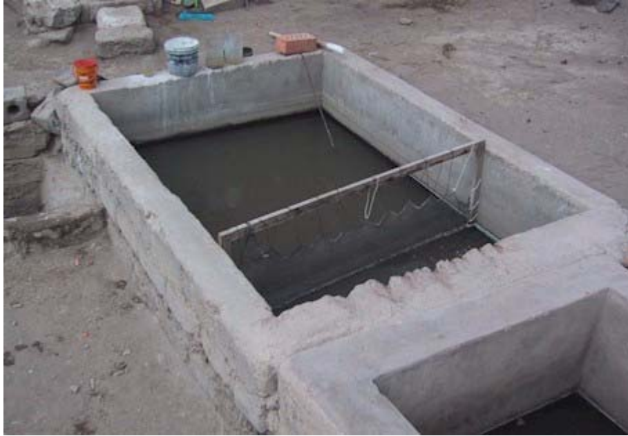
Figure 6.3: CBV Treatment Plant - First Tank with Screen
