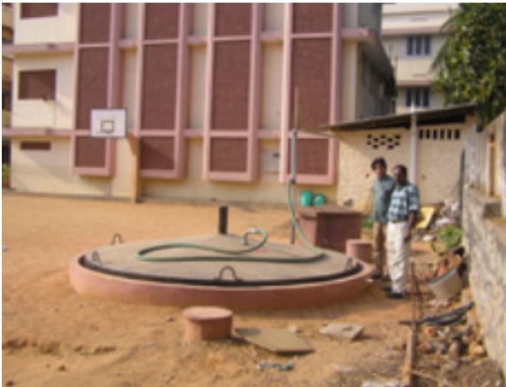
Figure 1: Institutional-scale biodigester at school in Trivandrum
