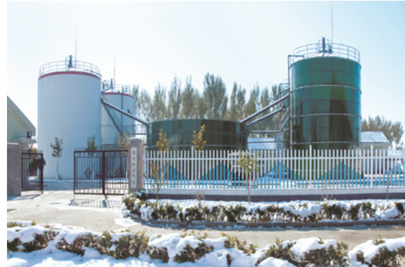
Large scale biodigester directly piping biogas to household cooking stoves
