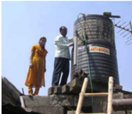
Roof installation of home-biodigester
