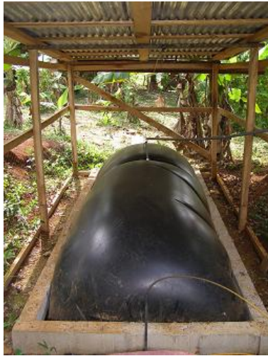
Polyethylene tube biodigester
