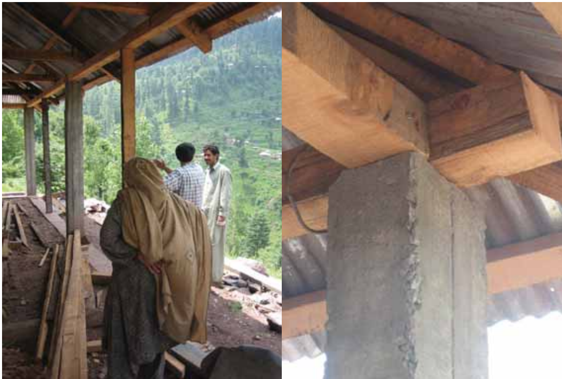
Picture 8. Eastern edge of residential area near the mountains. Sloped terrain. New construction site (after the earthquake).
