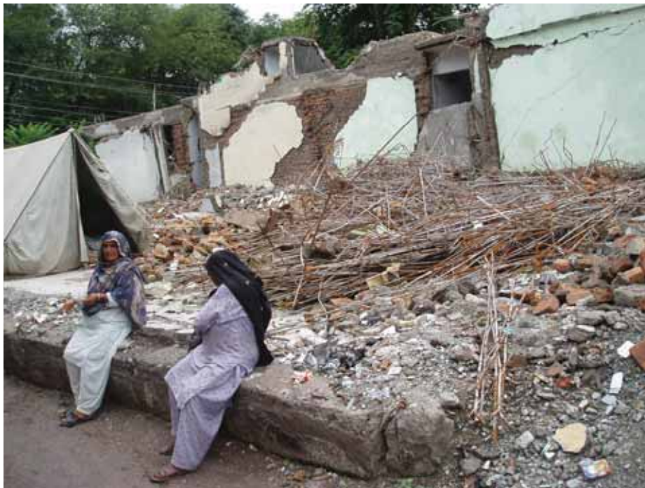
Picture 2. Old part of city near ancient ruins. Standard bricks. 30-70 years old. Original building was 3 stories tall; only parts of back wall remain. The metal rods were not part of the original building that collapsed. Flat terrain.
