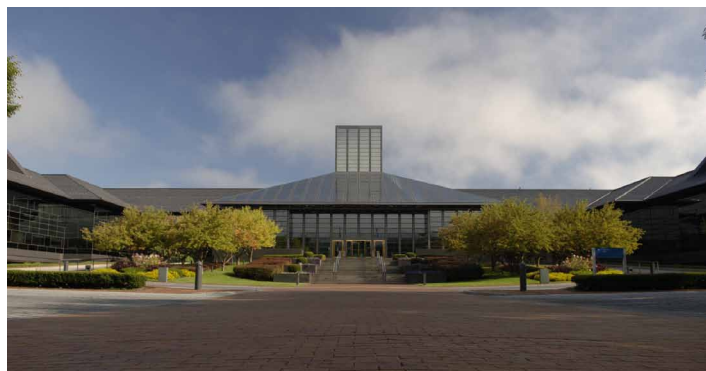
Corning Inc.'s headquarters building in Corning, NY.
