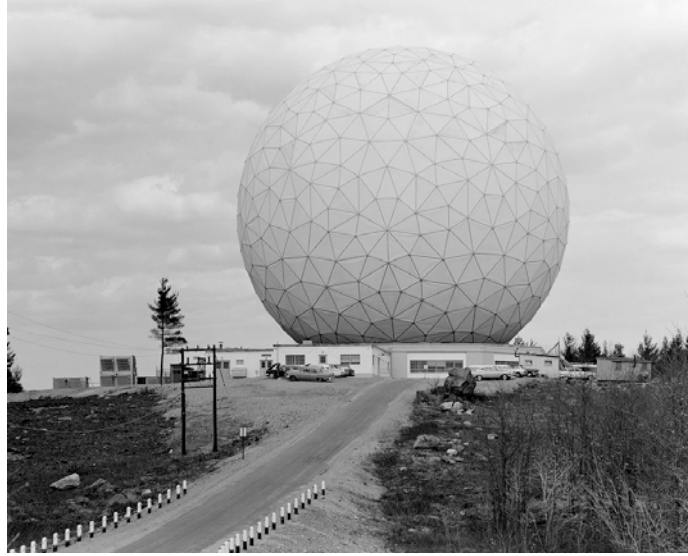
Figure 4: Lincoln Laboratory’s Haystack radar facility, completed in 1964. (Source: MIT Lincoln Laboratory.)
