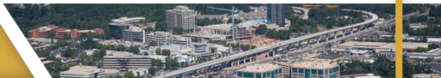
Tysons Corner Underconstruction | VDOT 2012
