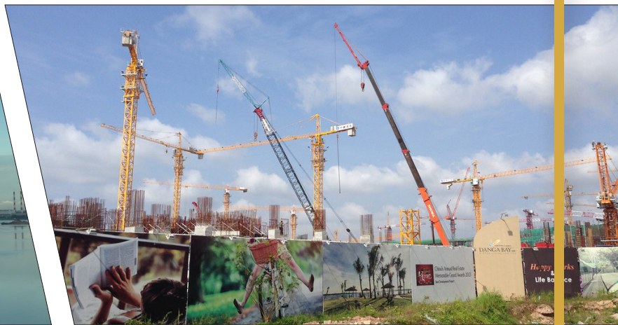
Construction in Johor Bahru | Andrew Binet 2015
