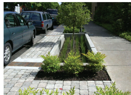
Linear Bioretention System. Plan shows how water cascades through a system of connected bioretention planters after each one fills to capacity
