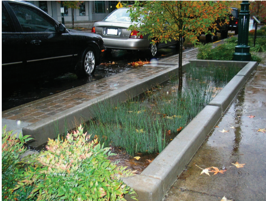
Integrated linear bioretention ponds can manage large volumes of ground runoff by linking many smaller components. Source: Kevin Perry, Bureau of Environmental Services, City of Portland, November 2005
