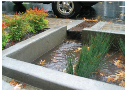
Linear Bioretention System. Plan shows how water cascades through a system of connected bioretention planters after each one fills to capacity
