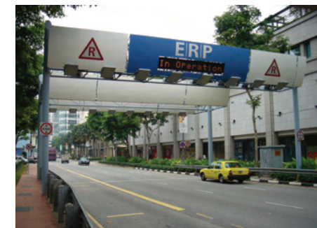
Gantries detect cars entering Singapore's congestion zone and charge drivers automatically (Source: "Electronic Road Pricing" 2007)
