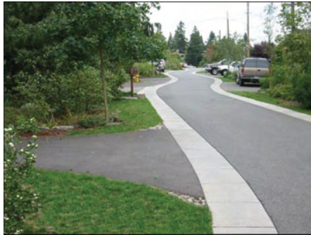
Seattle's SEA Streets utilizes simple swales to control runoff. Source: City of Seattle Public Utilities.
