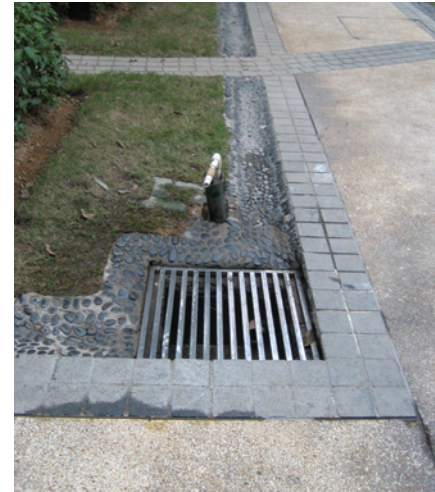
An example of Wonderland's current drainage system. Water flows off pathways directly into the municipal system. Source: Molly Mowery
