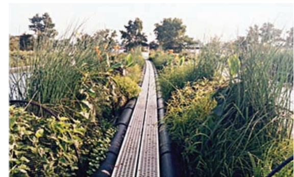
Floating rafts of 'engineered ecologies' > A rendering and a built example of Ocean Ark International's natural water quality system, the Restorer. Source: Ocean Arks International
