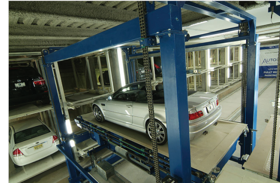
Automated Parking Garage by Stolzer Parkhaus > This high-efficiency garage allows for increased security, simplicity, and efficiency for both the parking customer and developer, despite the fact that the structure is underground. A customer can retrieve his car within three minutes. Source: New York Times.
