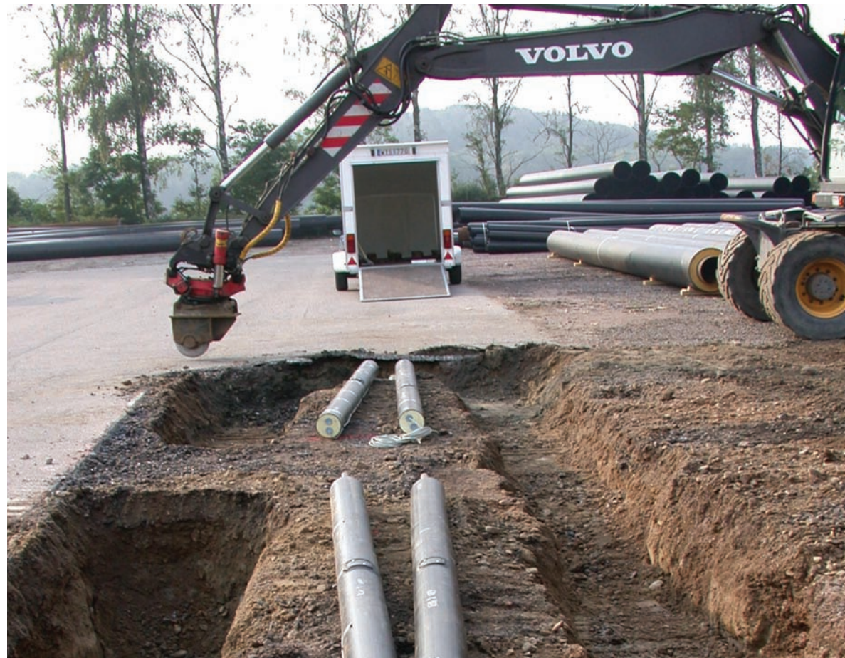
District Heating/Cooling Network Installation > Piping is installed for a district heating and cooling network in Sweden. Pipes must be heavily insulated and buried underground. Source: SP Technical Research Institute of Sweden 2008.
