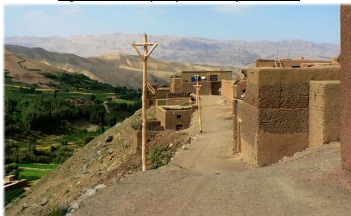
Figure 5: Electricity Project in Bamiyan Province
